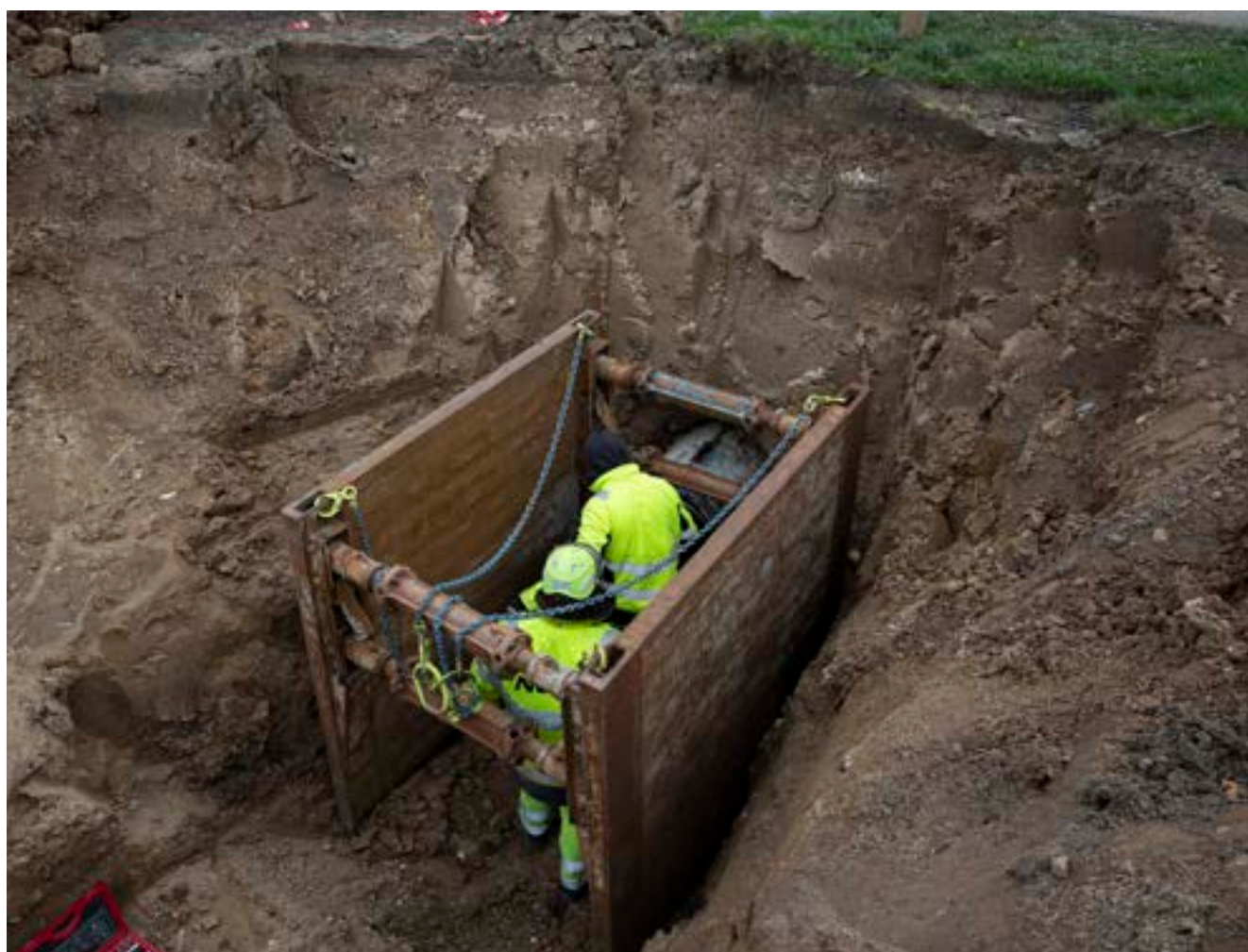
Underboring i Sengeløse
